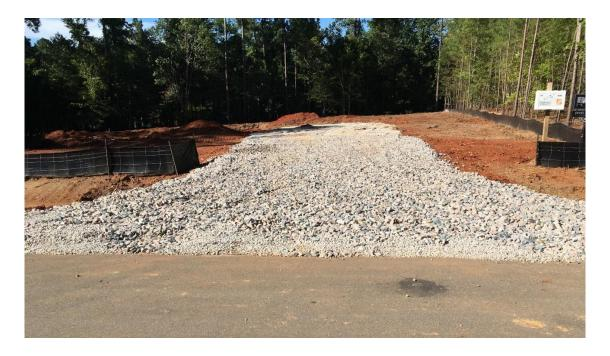
Construction entrances are often the most visible areas of a construction site to the public. Construction entrances provide an area where mud can be removed from tires prior to entering the public roadway. A well-maintained construction entrance reduces the amount of mud tracked off site, keeps roadways looking neat, improves public perception and complies with State and Wake County requirements.
